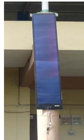
Fig. 8: Flexible PV (façade position)
